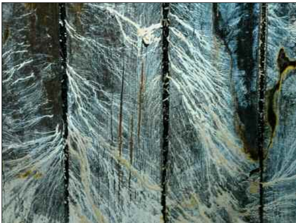
Figure 3. – Antrodia vaillantii , rhizomorphes (photo Protector Belgium).
