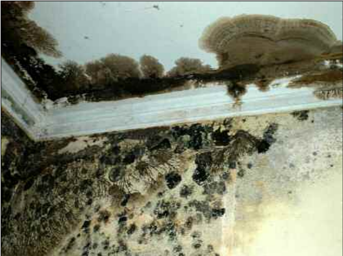
Figure 5. – Coniophora marmorata , carpophores et rhizomorphes (photo Protector Belgium).
