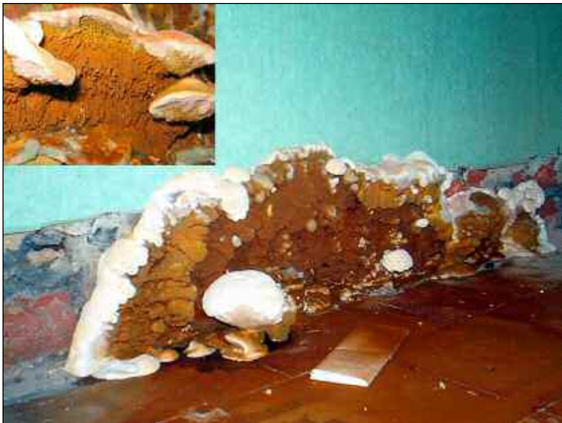
Figure 4. – Serpula lacrymans (mérule), carpophore et sporée (photo Protector Belgium).
